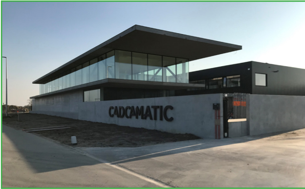
Atkore Vergokan Name: Cadcamatic Vertical Market: Industrial Products Used: Cable Trays & Floor Installations
