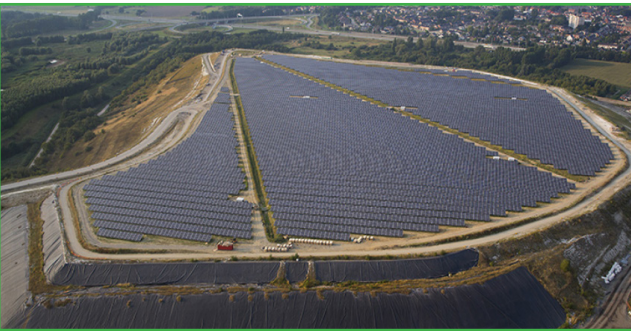
Atkore Vergokan Name: Gipsberg Vertical Market: Power & Energy Products Used: Wire Cable Trays
